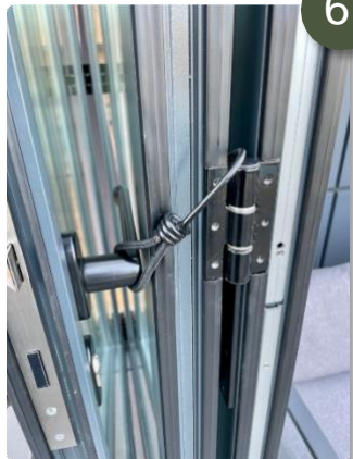
Protect against gusts of wind with expander hook (you will find it in the cutlery drawer)
